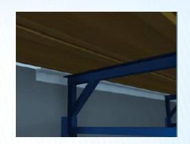
Once the grooved angles are installed around the perimeter, formworks are moved to the upper floor.
