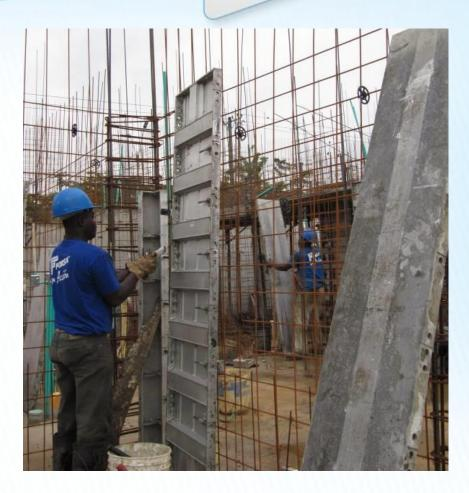
In height, it is recommended to start by the internal faces of walls facades
