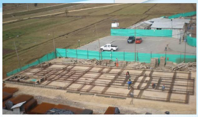
Accurately locate reinforcing steel, hydraulic, sanitary and electrical networks.
